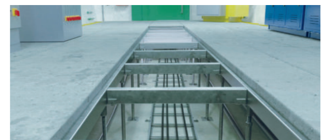
Steel frame with C-profiles
