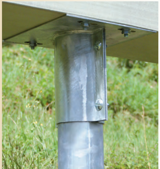
Post head adjustable in 2 directions
